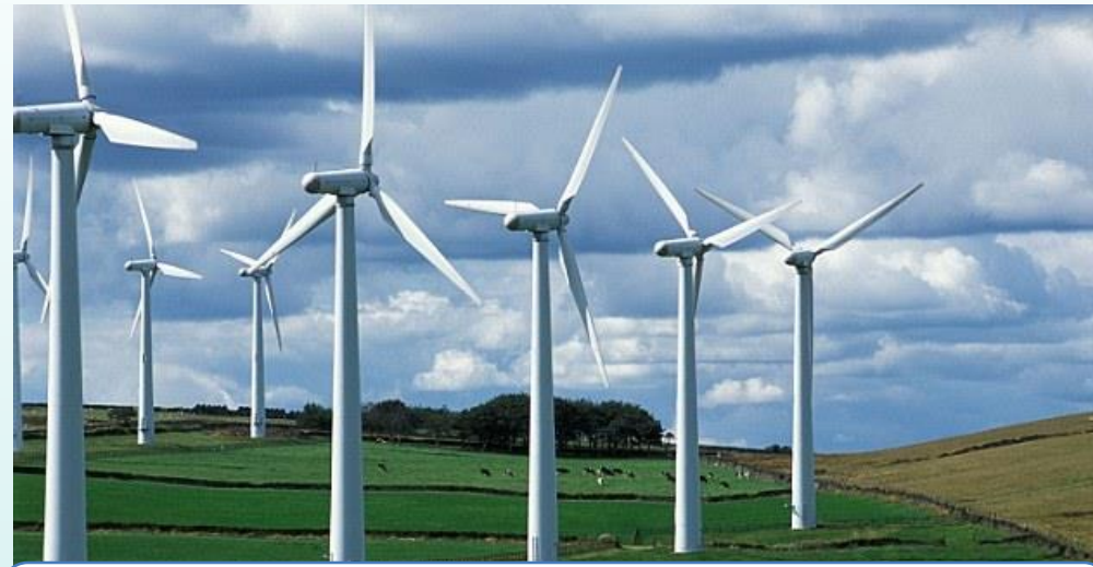
Wind plants use energy from wind and convert it into electricity
